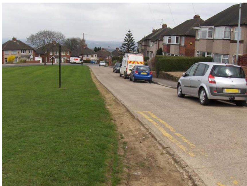
Evidence of verge running on Hayfield Crescent
